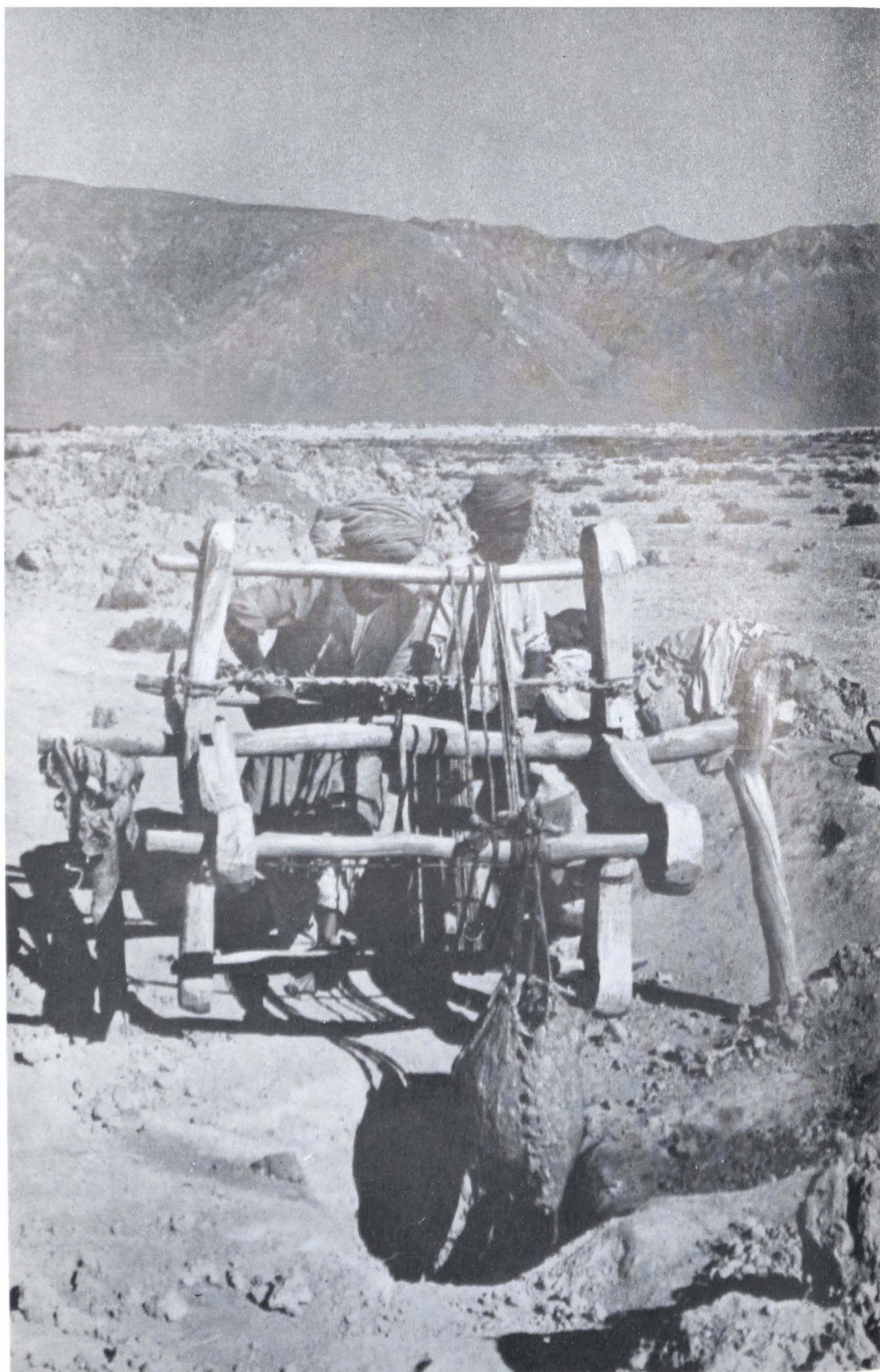
Curing a 'kanat' of its mud (Chapter 16)
